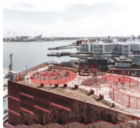
Multi use parking facilities with high quality architectural design. Park n' Play, Copenhagen by Jaja Architects. Image: R. Hjortshoj.
