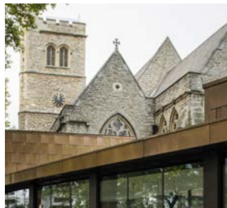
Sympathetic refurbishment and extension to a listed heritage asset. Garden Museum Extension by Dow Jones Architects. Image: Anthony Coleman.
