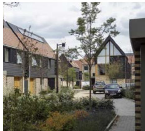
Parking, including car club spaces, integrated into public realm. Parking example at Great Knieghton by Proctor and Matthews Architects. Image: Tim Crocker.
