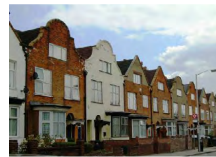
Photo 48. Terraced houses on Melfort Road
