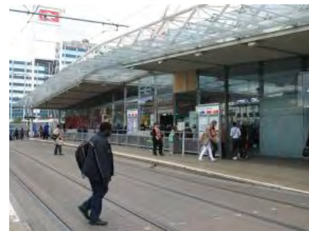
Photo 48. East Croydon Station
