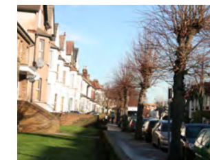
Photo 24. Larger residential terraces
