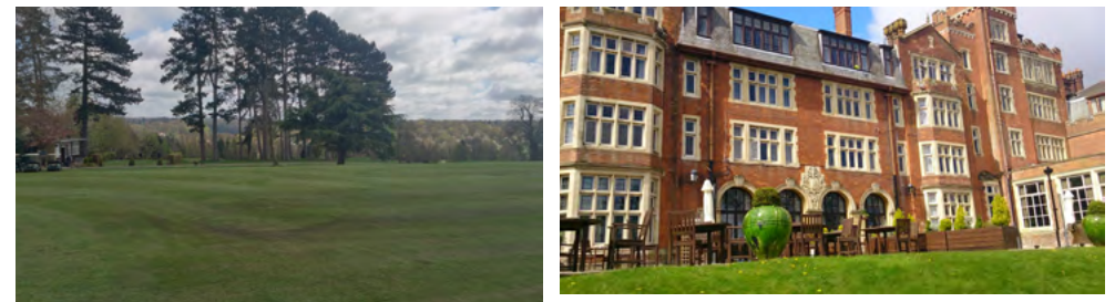
Photo 10. Large Victorian houses in the East India Estate Conservation Area Photo 11. Detached houses in Whitgift Estate
