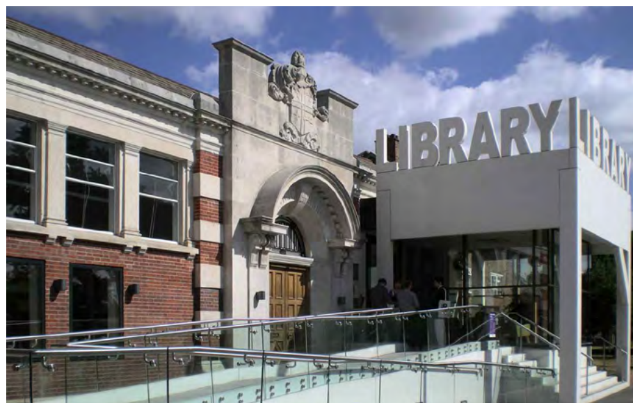
Photo 46. Thornton Heath Library
