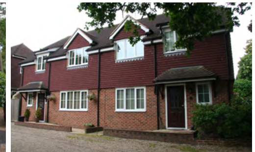
Photo 16. Compact houses on Upper Shirley Road
