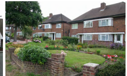
Photo 14. Maisonettes on Cheston Avenue Estate
