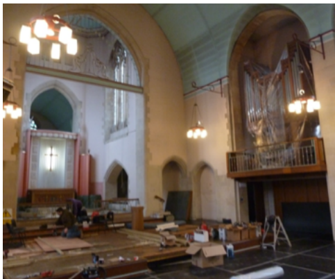
Getting underway; work on the new platform in the nave
