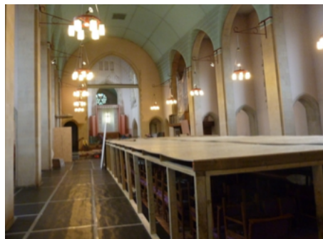
Covering everything up, ready for the work to get going
