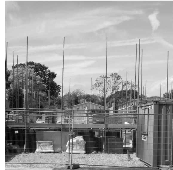
Not 10 flats but 1 Archdeacon's home Building work starts on Sefton Road
